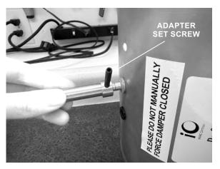
3. Install the DDC-S 5/16" to 1/2" shaft adapter onto damper shaft. Align set screw with desired minimum position setpoint and tighten it down.
