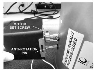
4. Align anti-rotation pin and install the HD-MOTOR-RR onto the damper shaft. With damper blade in open position, tighten down set screw.
