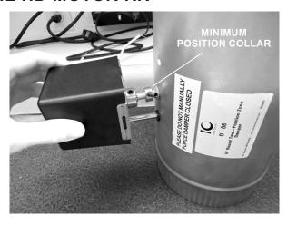
2. With the damper spring returned open (blade in open position), loosen the set screw on the actuator and minimum position collar. Remove actuator and collar.
